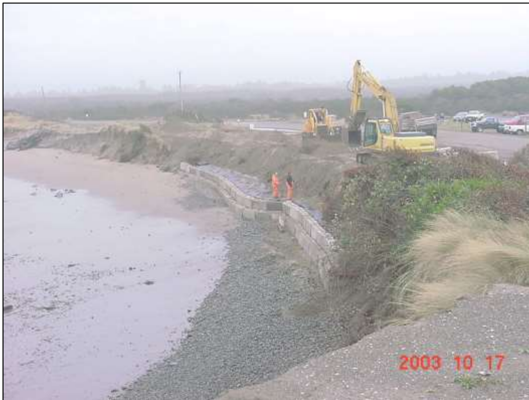
Figure 7-11 Emergency Dune Protection Constructed at Half Moon Bay, Westport, October 2003
