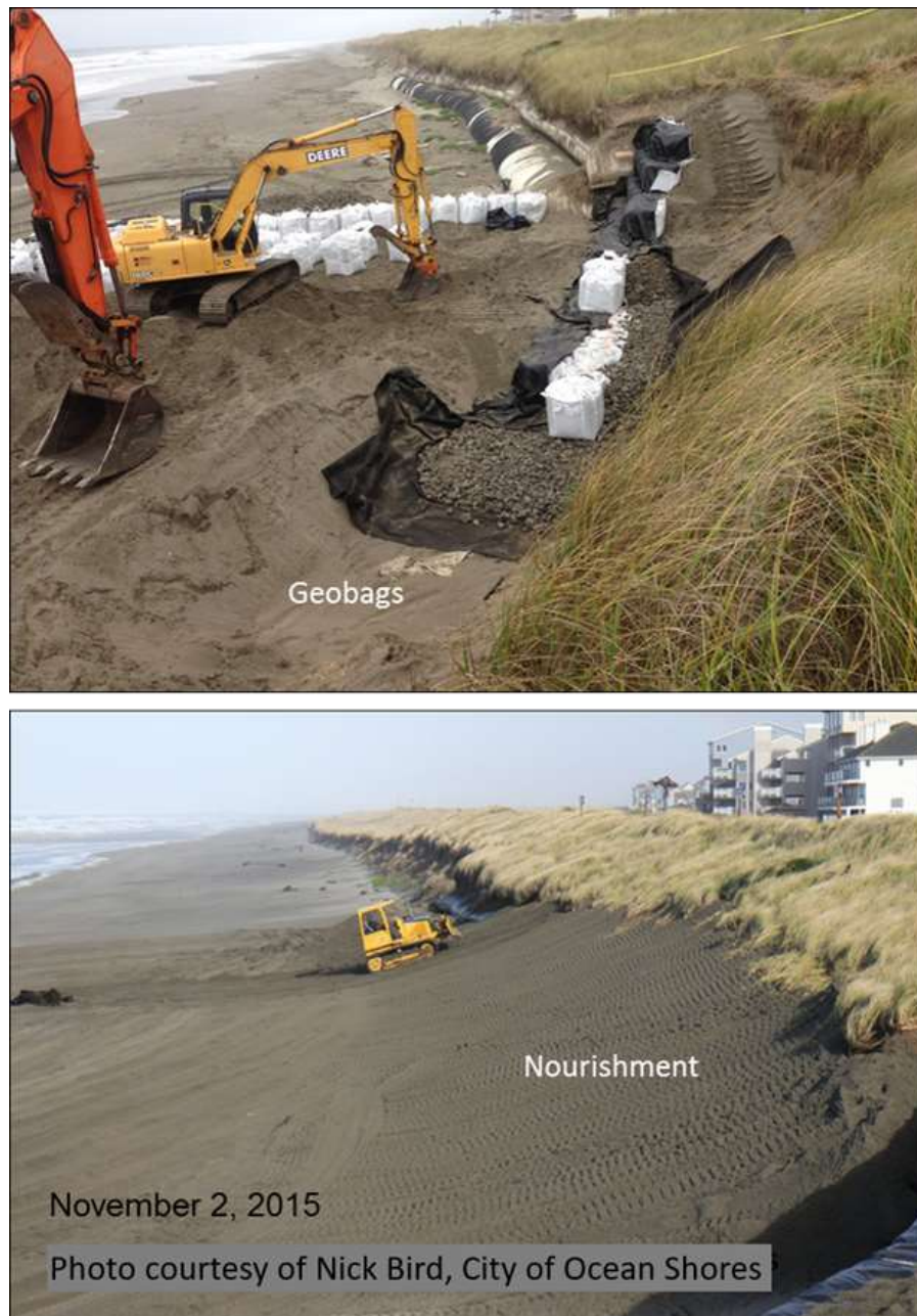
Figure 7-19 Photos of Geobags and Dune Nourishment at Ocean Shores in November 2015
