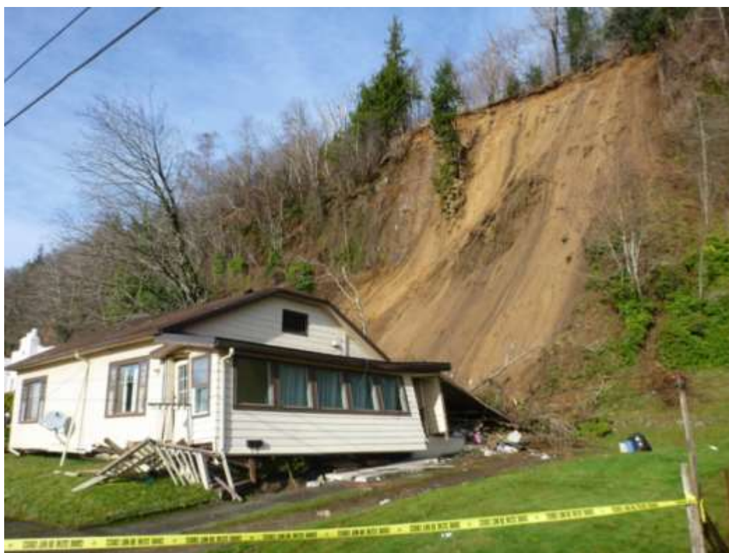
Figure 9-7 Structure Impacted by January 2015 Landslide Event
