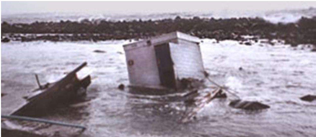
Figure 10-21 Restroom at North Beach Destroyed by Winter Storm Waves
