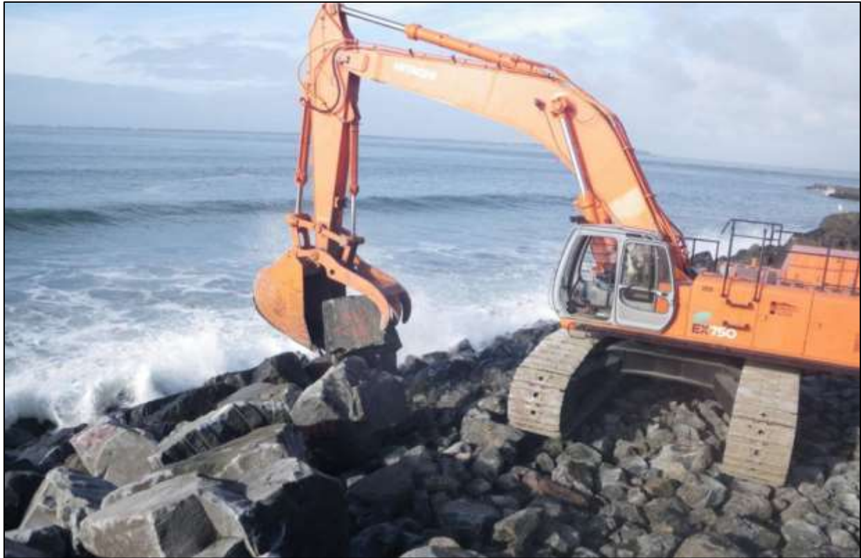
Figure 7-13 Photo of Point Chehalis Revetment Repairs in 2013 from Michalsen and Brown (2015)
