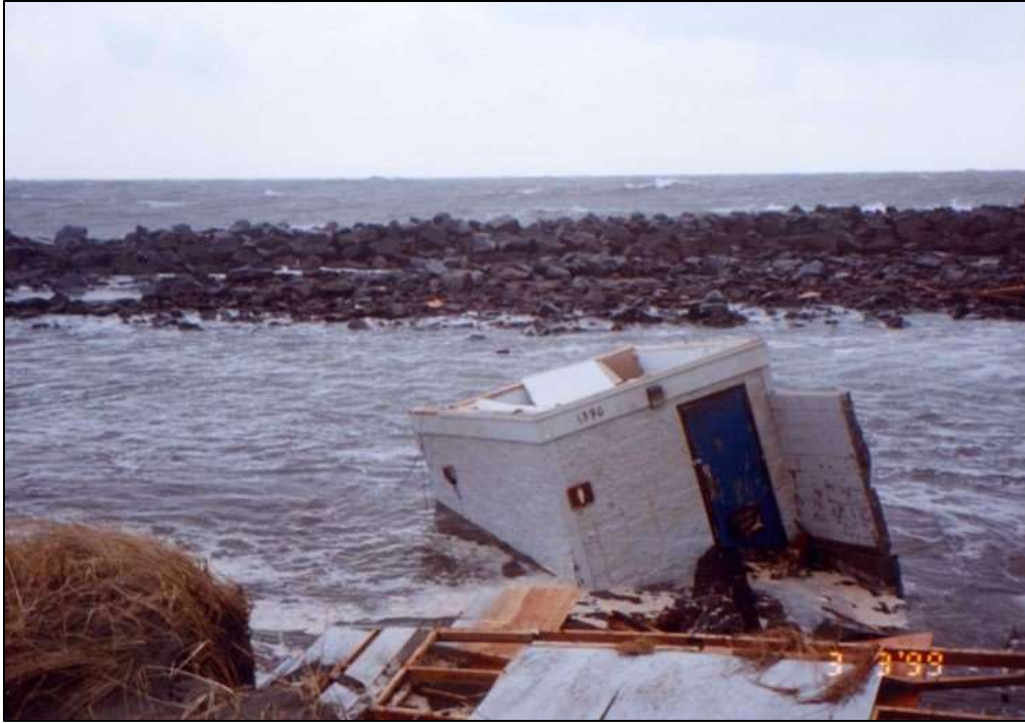
Figure 7-16 Flooding and Erosion of the Ocean Shores Public Restroom During March 1999 Storm
