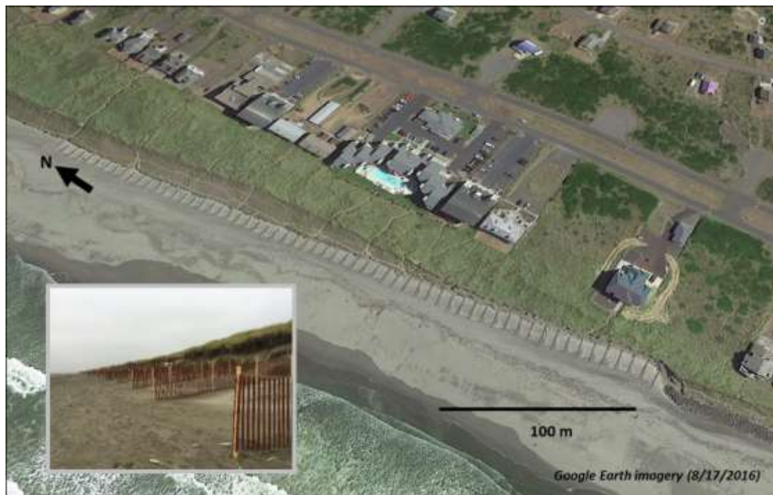
Figure 7-22 Sand Fences Installed North of the Ocean Shores Rock Revetment in 2016
