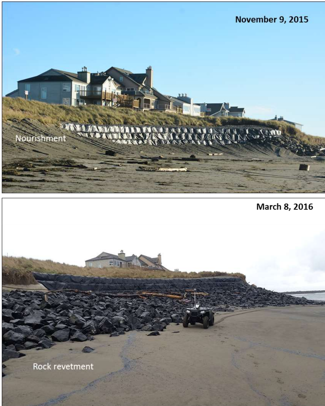
Figure 7-20 Geobags Nov. 2015 and Rock Revetment Installed in Front of Geobags Winter 2016
